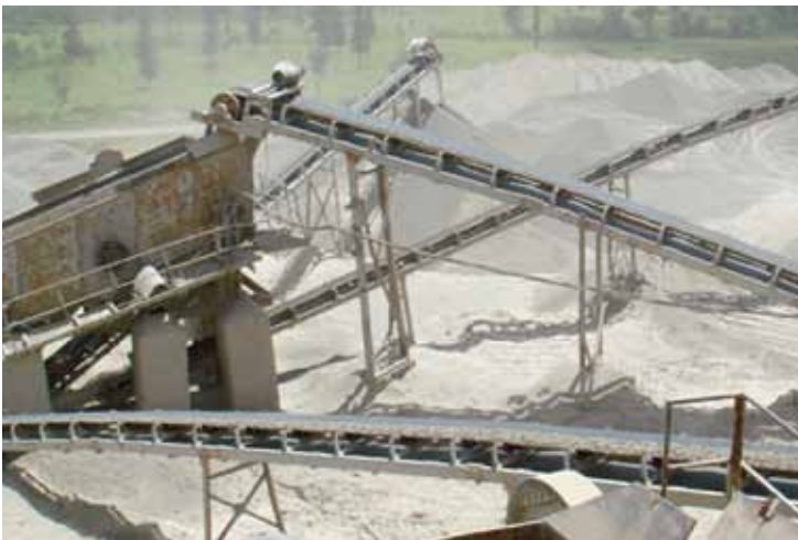
Fig. 2.9. Crusher at Kirima Quarry, Molo
