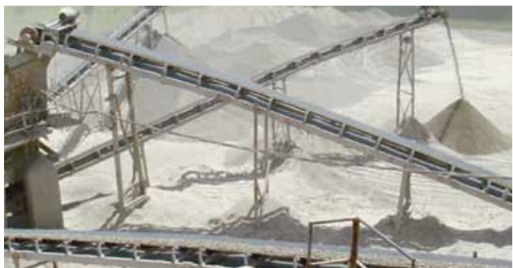
Fig. 3.3. Post-dust suppression, Kirima Quarry
