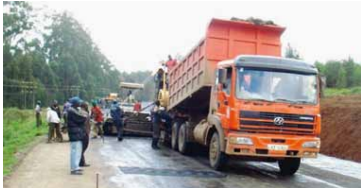
Fig. 2.15. Bitumen application, Nakuru-Mau Summit Road
