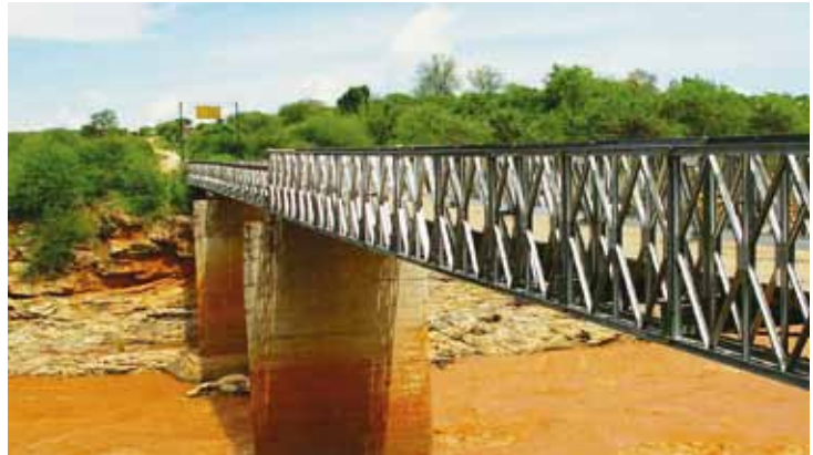
Fig. 2.17. Bailey bridge crossing the Tana River
