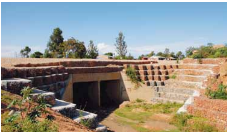
Fig. 1.3. Sondu River and embankment/bridge protection works
