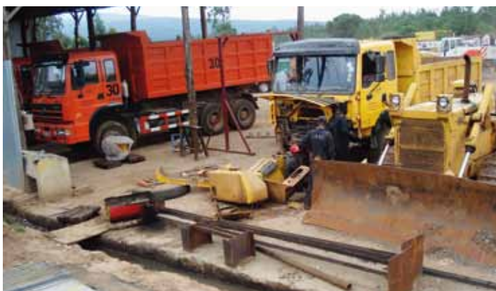
Fig. 2.1. Camp workshop with trenches to retain/redirect water runoff
