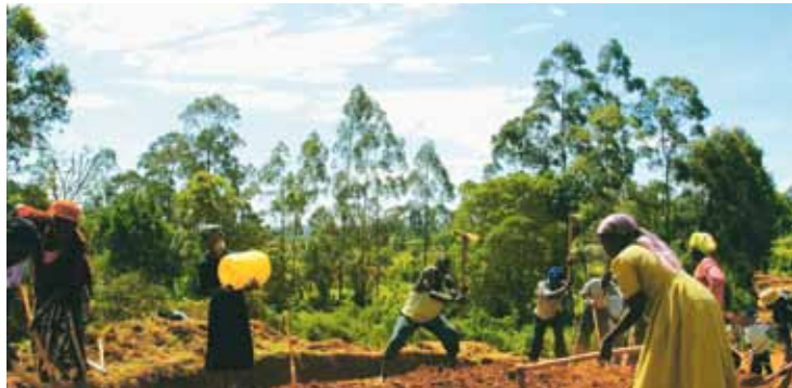
Fig. 7.1. Labour-based construction, rural road, Nyanza
