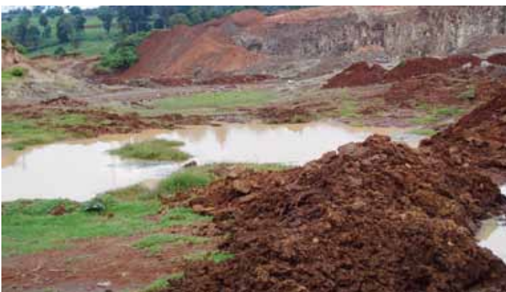
Fig. 2.8. Unreinstated borrow pit, Mau Summit
